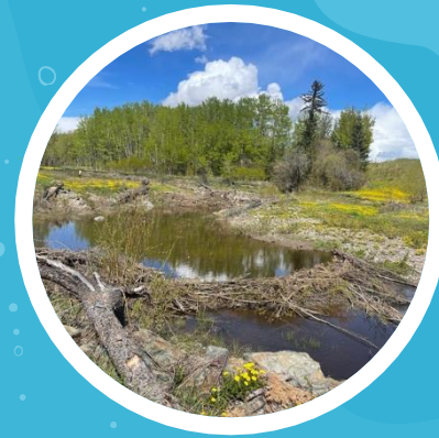
Completed BDA, Knight Creek
