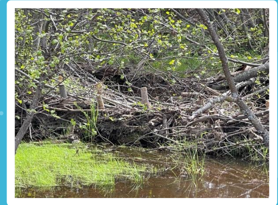
Completed BDA, Knight Creek
