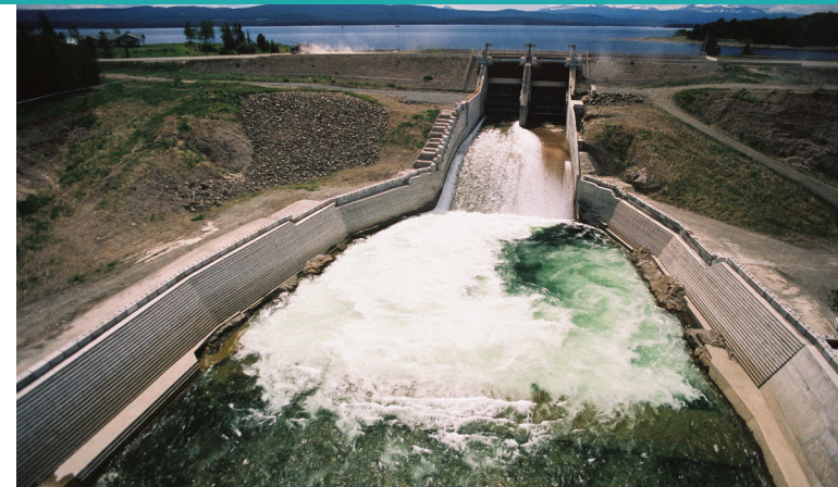
Skins Lake Spillway releases water from the Nechako Reservoir into the Cheslatta system, which flows into the Nechako River.
