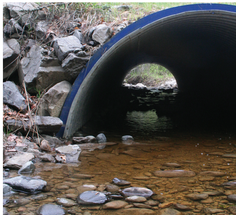
LEFT MIDDLE: Shown here is a new culvert at a road crossing on Murray Creek. The old culvert prevented fish from moving upstream during certain times of the year when the flow was low or very high. The new culvert now allows for fish passage. This is one example of a stream rehabilitation project that NEWSS undertakes to improve fish habitat.
