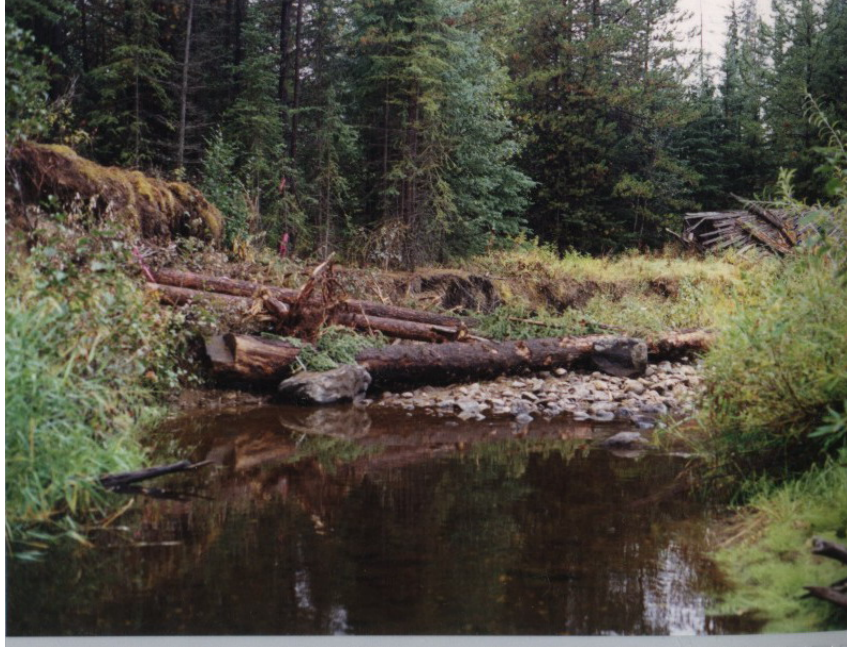
Corkscrew Creek, Reach 5 (site 98-05) at time of construction.
