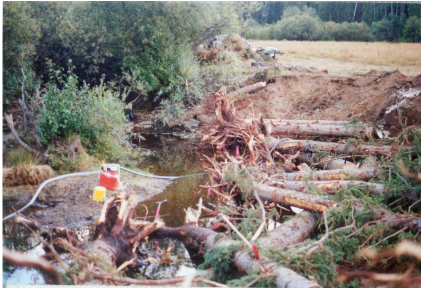
Corkscrew Creek, Reach 4 (Site 98-02) during revetment project. Photo taken upstream.
