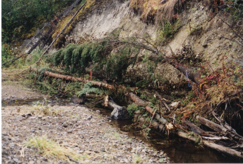
Corkscrew Creek, Reach 5 (Site 98-02) at time of construction of stabilizing structure.
