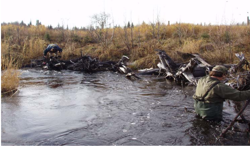
Corkscrew Creek, Reach 4 (Site 98-02) following revetment project in 2005. Photo taken upstream.
