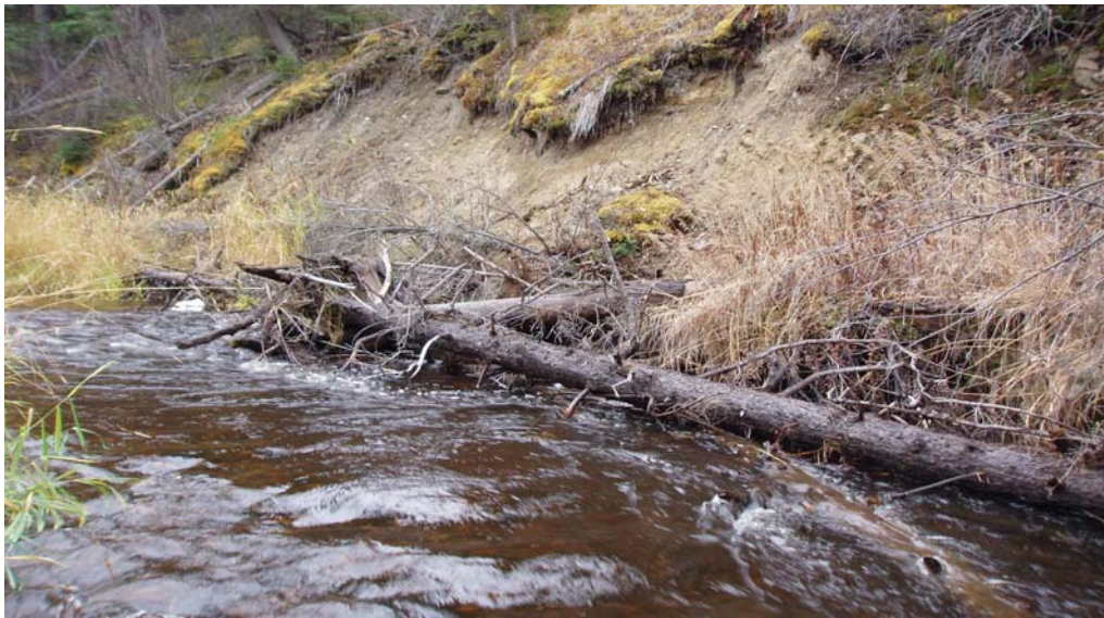
Corkscrew Creek, Reach 5 (Site 98-02) as of 2005. Note established grasses as indicator of stabilization.
